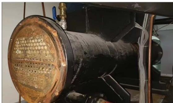
Figure 1. Scaling in condensers
