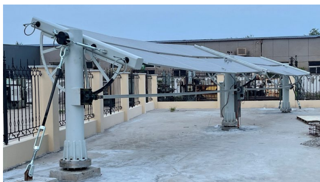
Figure 22. The Tracking flexible photovoltaic system 图 22. 跟踪式柔性光伏系统
