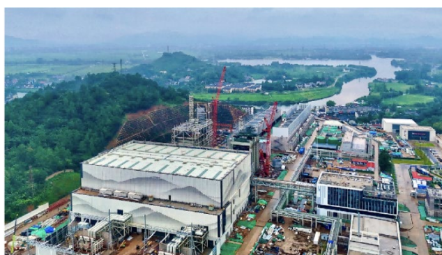
Figure 1. An aerial view of the Anji gas turbine plant in Zhejiang 图 1. 浙江安吉燃气轮机厂区远景
