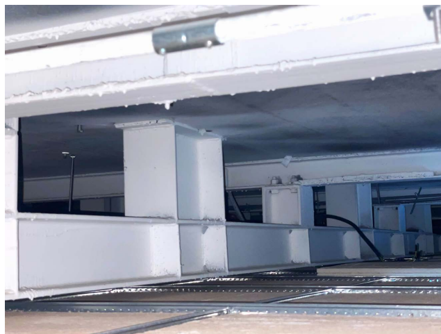
Figure 1. Open web truss combined floor cover without chord 图 1. 无上弦空腹桁架组合楼盖
