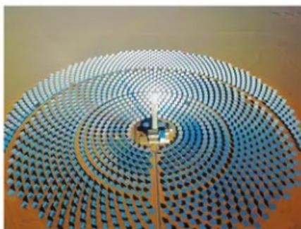
Figure 1. Tower solar thermal power generation
