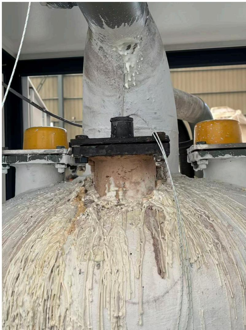
**Figure 7.** The molten salt splashes onto the tank body through the installation opening of the temperature measurement device
