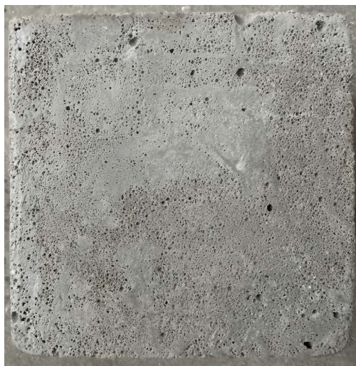
Figure 4. Untreated specimen surface
