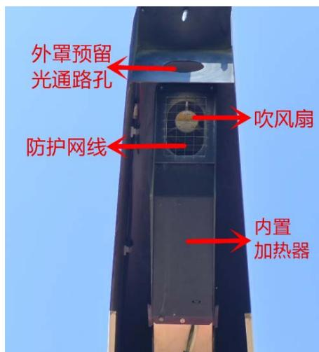
Figure 3. TR30LED receiver emission window structure diagram
