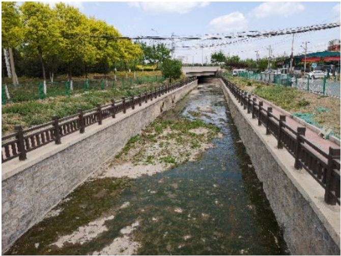
Figure 1. Current situation of the river channel 1 图 1. 河道现状 1
