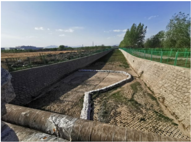
Figure 2. Current situation of the river channel 2 图 2. 河道现状 2
