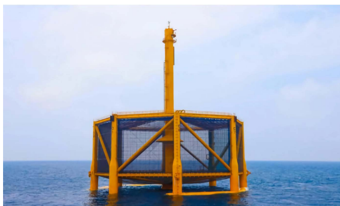
Figure 2. Far-reaching marine aquaculture equipment facilities using UHMWPE rope nets
