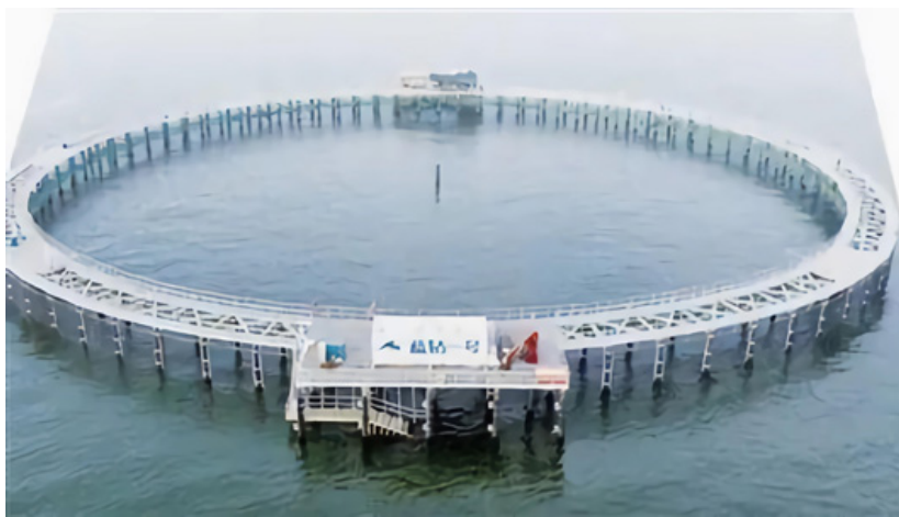
Figure 5. Double circumference pipe pile type large fence breeding facilities 图 5. 双圆周管桩式大型围栏养殖设施
