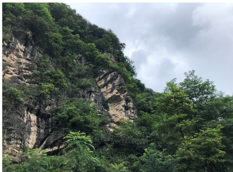
Figure 2. Photos of dangerous rock mass W5
