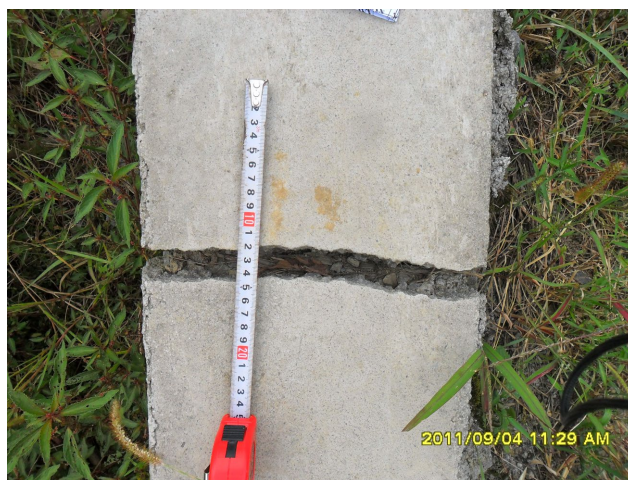
Figure 5. Cracked retaining wall at the rear edge of the landslide 图 5. 滑坡后缘挡土墙开裂
