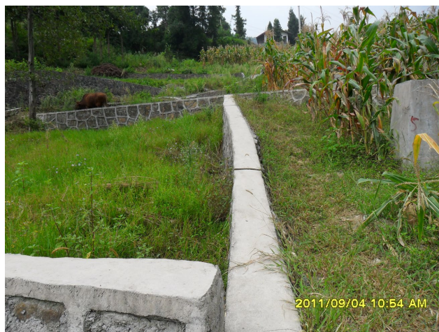
Figure 6. Subsidence of the retaining wall at the rear edge of the landslide 图 6. 滑坡后缘挡墙下挫
