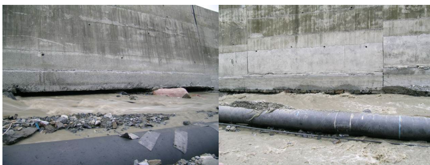
Figure 2. Photo of the scoured foundation of the retaining walls on both sides of the river channel
