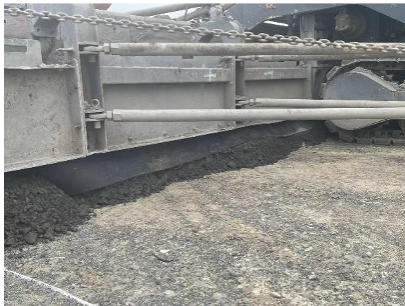
Figure 7. The baffle of the paver 图 7. 摊铺机挡板
