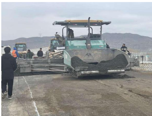
Figure 5. Aggregating hopper of the paver 图 5. 摊铺机集料斗
