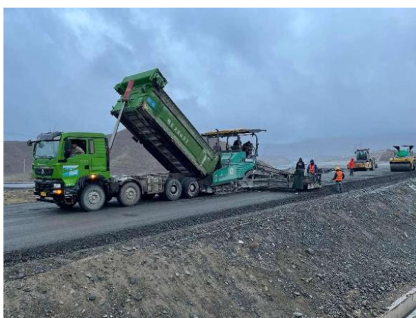
Figure 4. The material carrier pours the material into the paver 图 4. 运料车向摊铺机倒料
