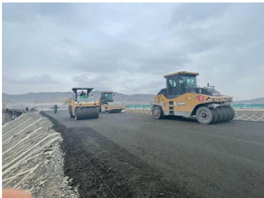
Figure 11. Combined rolling 图 11. 联合碾压
