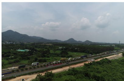
Figure 1. Live view of the Kaiyang expressway expansion and renovation project 图 1. 广东省开阳高速改扩建工程实景
