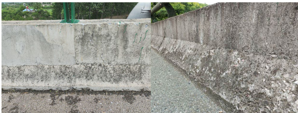
Figure 1. Concrete guardrail without protective coating
