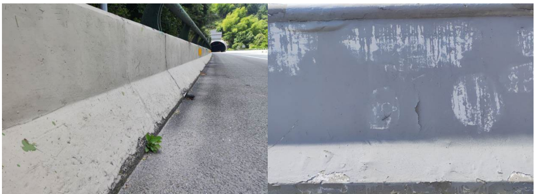
Figure 7. Acrylic polyurethane coating (left), fluorocarbon coating system (right) 图 7. 丙烯酸聚氨酯涂料(左)、氟碳体系涂料(右)
