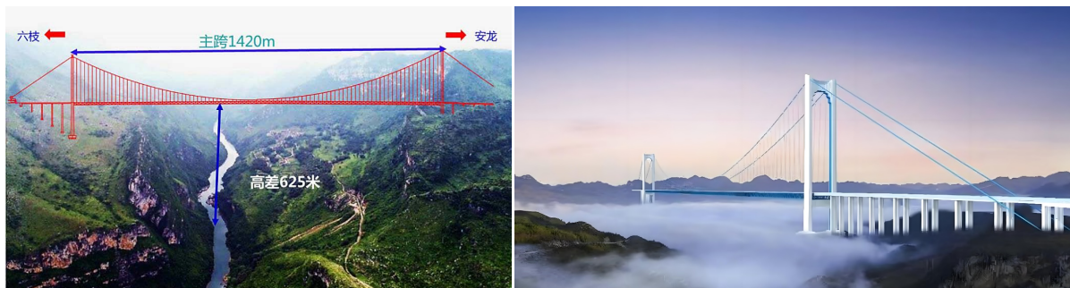
Figure 4. Schematic diagram of the design and completion of the Huajiang Gorge Bridge 图 4. 花江峡谷大桥设计及竣工示意图
