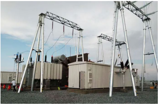
Figure 1. Energy saving cabinet equipment for photovoltaic power station collection line 图 1. 光伏电站集电线路节能柜设备
