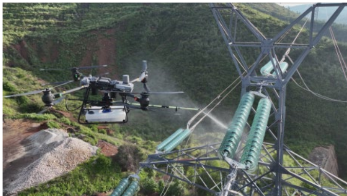
Figure 4. Drone cleaning 图 4. 无人机清洗
