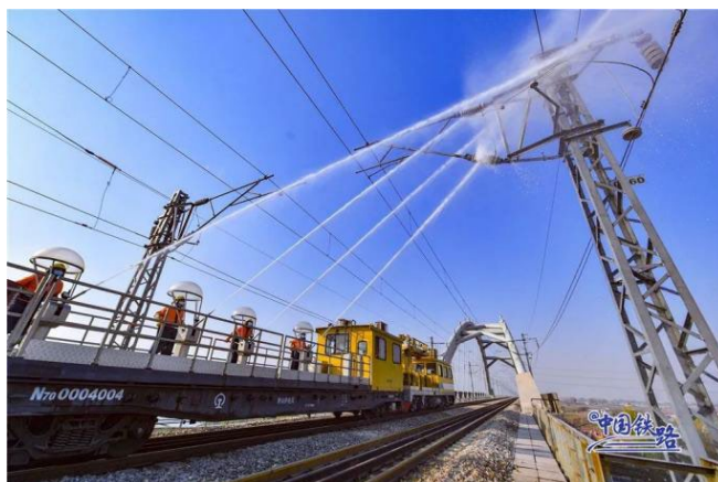
Figure 7. Water flushing operation scenario
