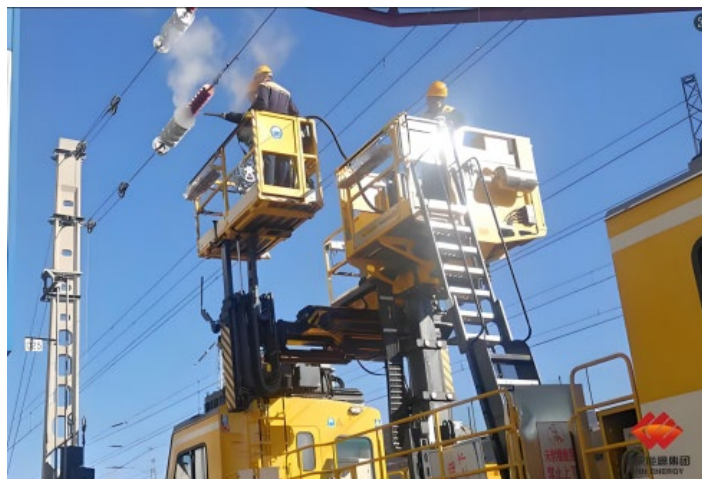
Figure 3. Dry ice cleaning (assisted by lifting platform)
