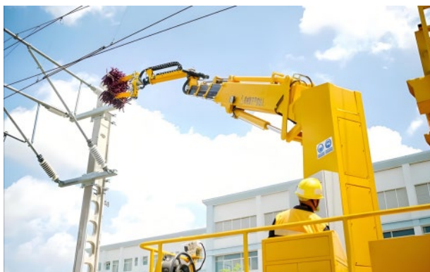
Figure 2. Large robotic arm assisted cleaning 图 2. 大型机械臂辅助清洗
