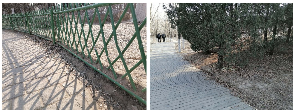
Figure 2. Sediment deposition at the bottom of the hillslope without understory grass cover (left) and with understory grass cover (right)
